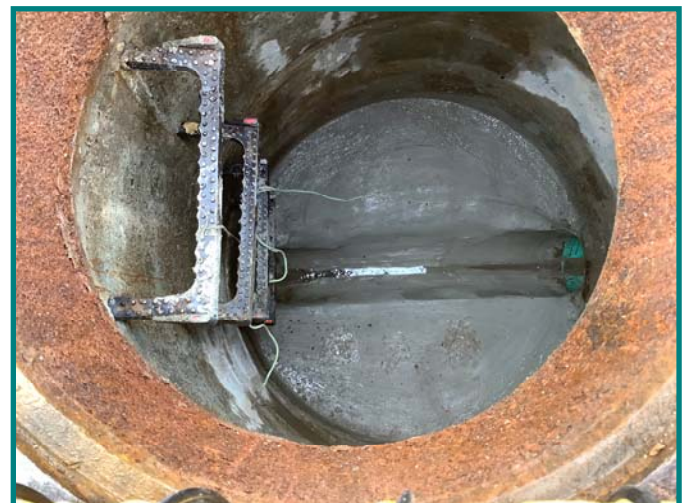
Repaired Manhole Channel
