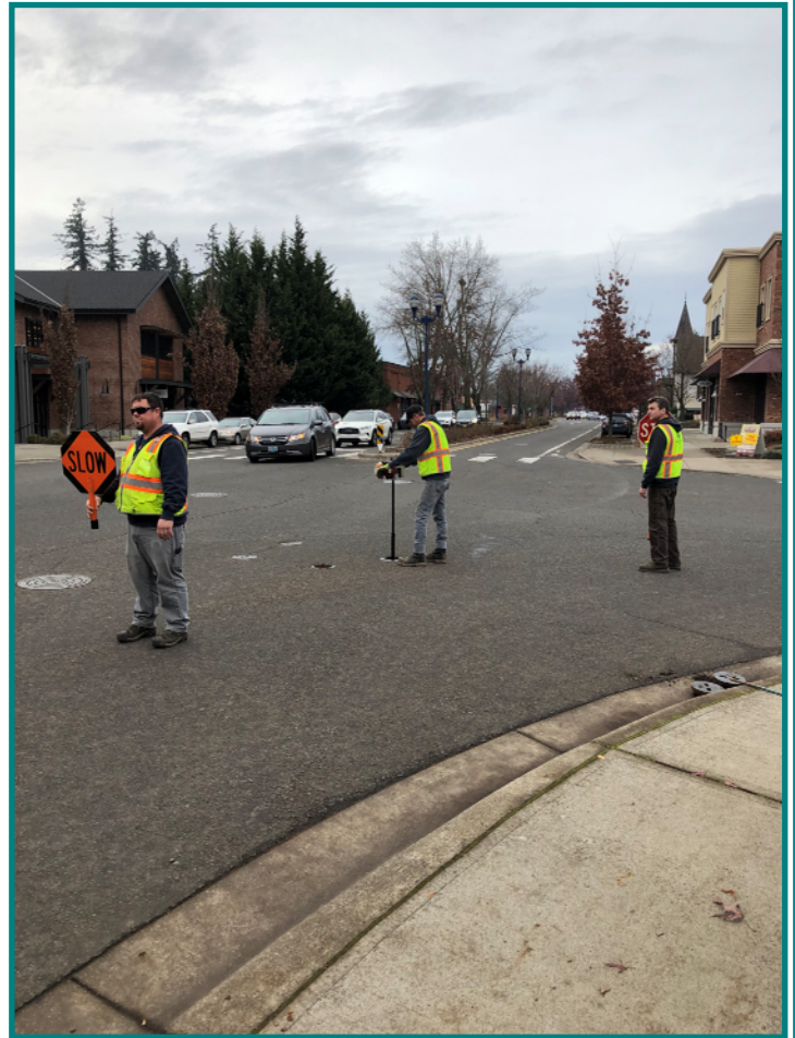
Chad Whiting & Paul Walker — Work Zone Flagging
