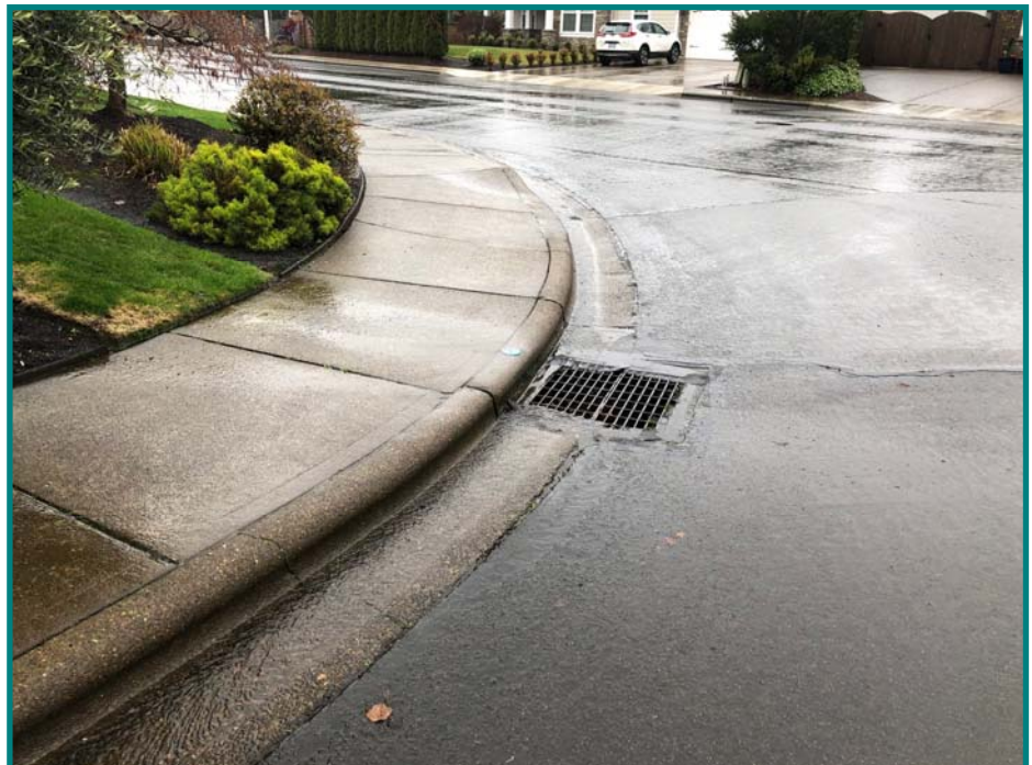
Same location after staff cleared the debris.
