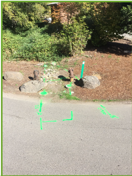
Showing the layout of the pipes
