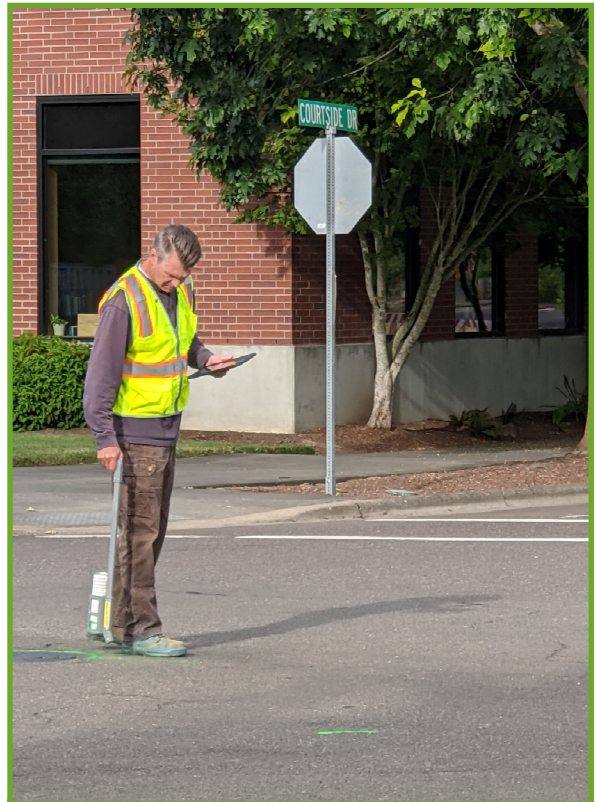
Paul Walker marking sewer lines
