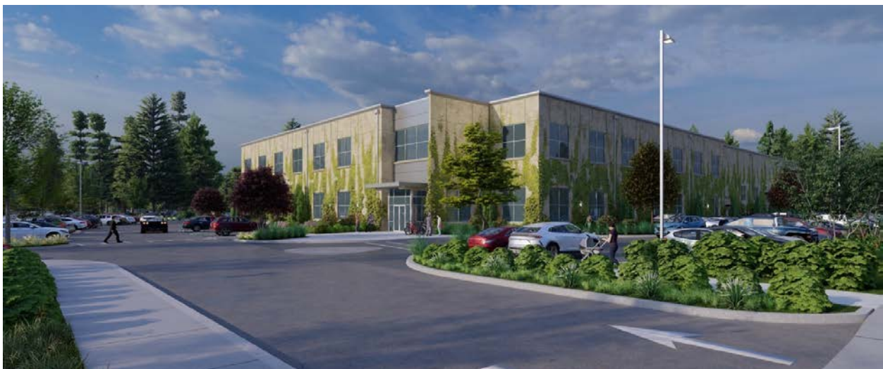
The proposed W5 hi-tech industrial building "shell" in morning light off SW Boeckman Road.
