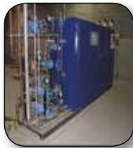
**Step 3 – Ozonation:** Clarified water from Actiflo™ is disinfected with ozone, an extremely powerful oxidizer which kills pathogenic organisms and breaks down taste and odor compounds.
