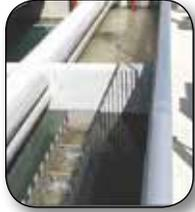
**Step 2 – Enhanced Coagulation, Sedimentation:** Raw water is treated with a coagulant and enters the Actiflo™ process, which quickly removes turbidity and other contaminants.
