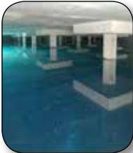
**Step 5 – Secondary Disinfection & Storage:** Filtered water is treated with chlorine which protects the water as it travels through the distribution system to City reservoirs.
