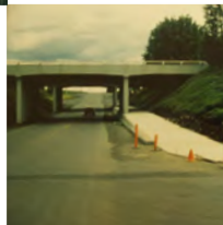
LEFT In 1983, a sidewalk was added to the original narrow I-5/Wilsonville Road interchange.
